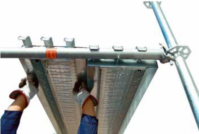
14 • erecting metal ledger planks
