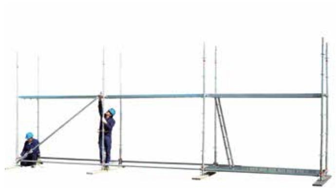
17 • erecting diagonals
