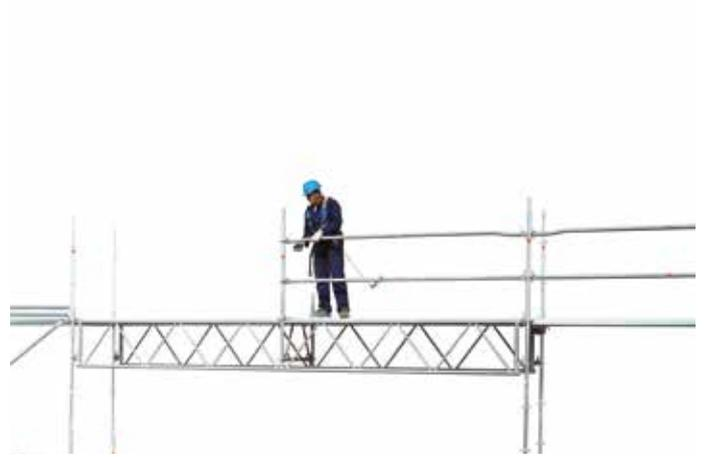
52 • erecting carriage beam guard rail
