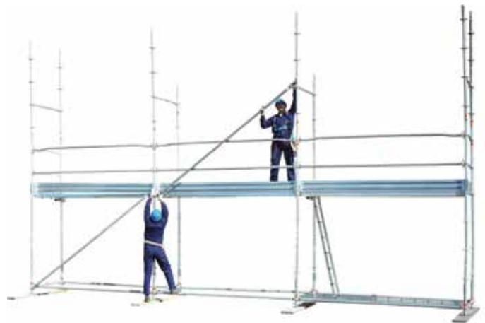
35 • erecting diagonals every 4 fields per floor
