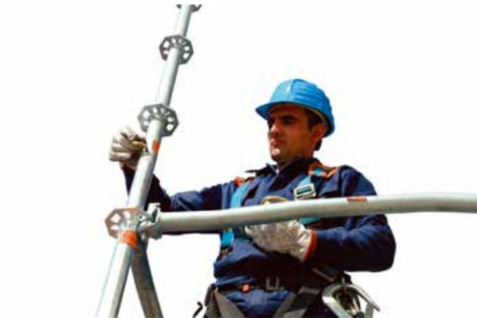
32 • inserting spigot pin connector
