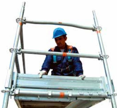
26 • erecting side fencing structure
