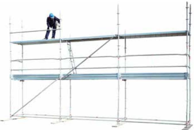
39 • erecting level 2 guard rails
