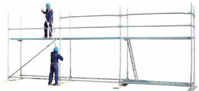
24 • erecting level 1 guard rail
