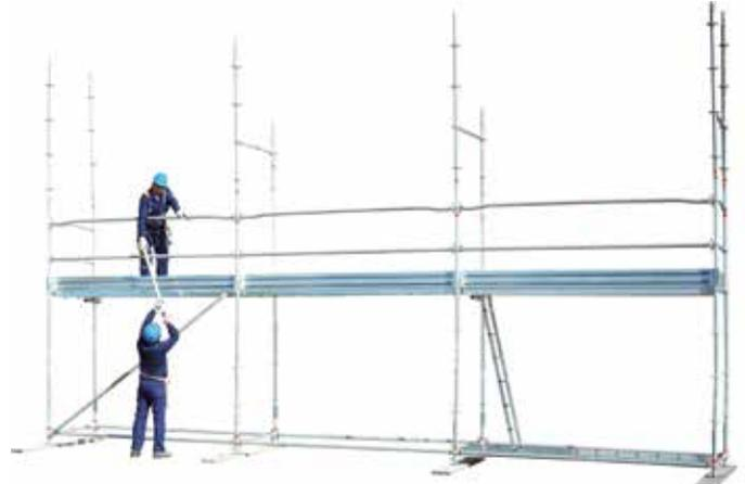
34 • erecting level 2 ledgers and guard rails
