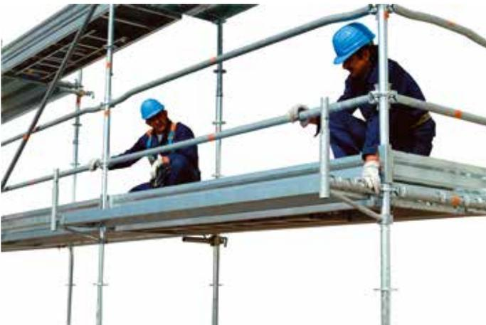
45 • inserting the wedge
