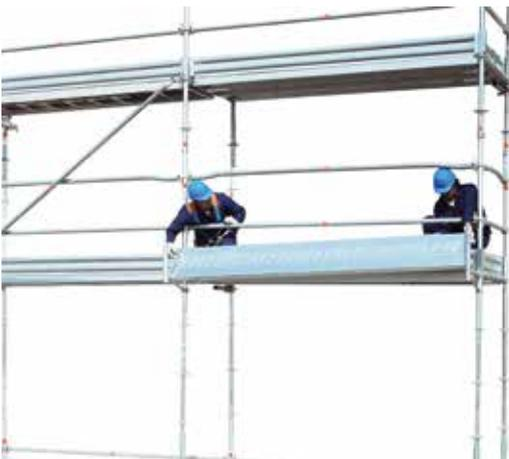
44 • erecting overhanging plank
