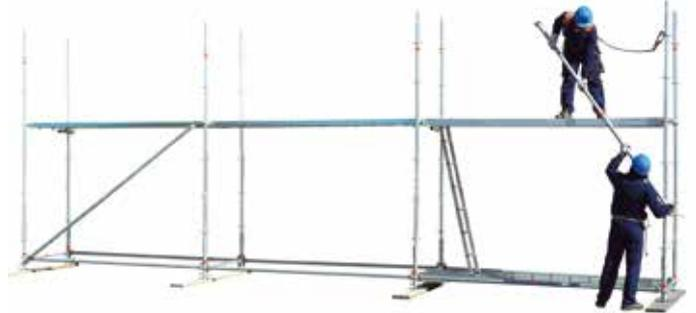
22 • erecting level 1 guard rail
